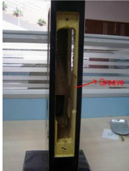
2. Screw the lock body in the lock hole and test if the latches can stretch freely.
