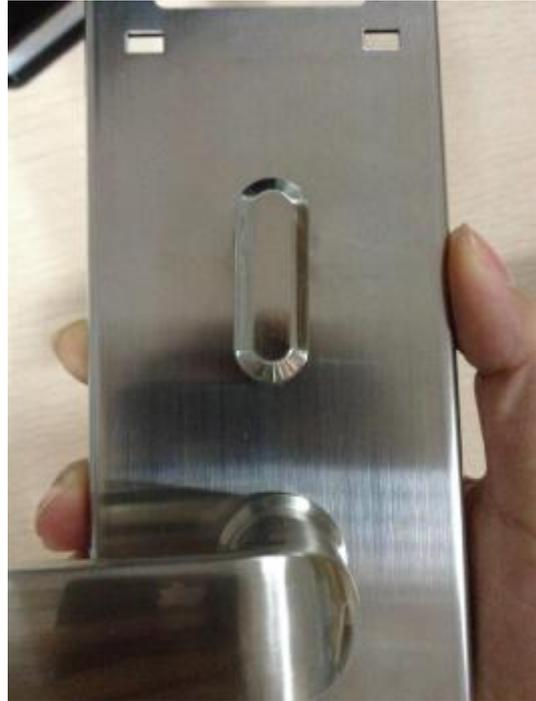
6. Connect the flat cables. Screw the four face plate fixed screws.
