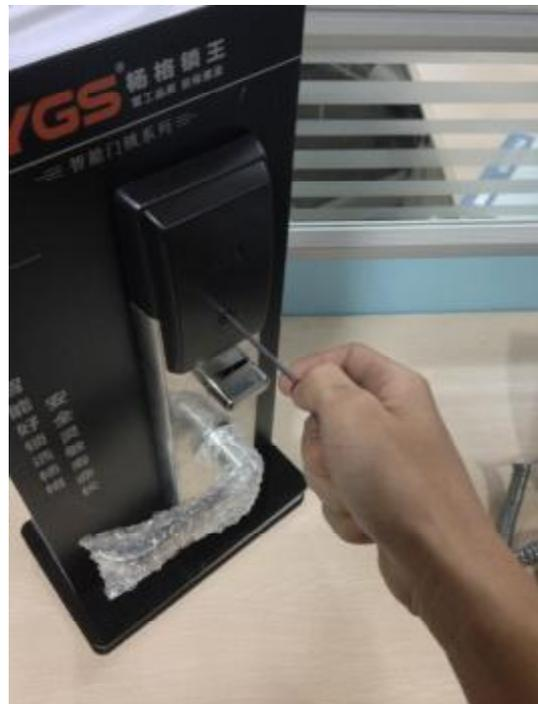
7. Check the lock installation by reading Engineering Card. If the lock can be opened, the installation is correct.
